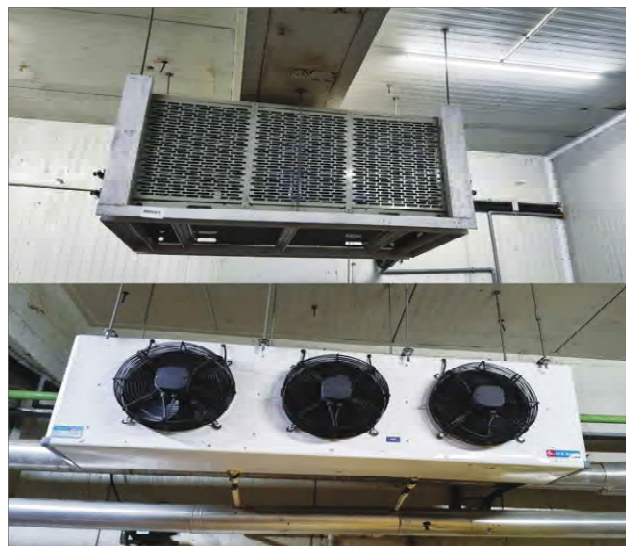
Dahi Incubation Room Indoor & Outdoor Unit worked as Heat Pump
